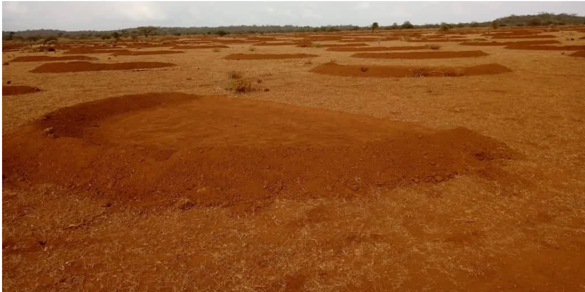
Figure 7: Bunds dug in Ilchalai
