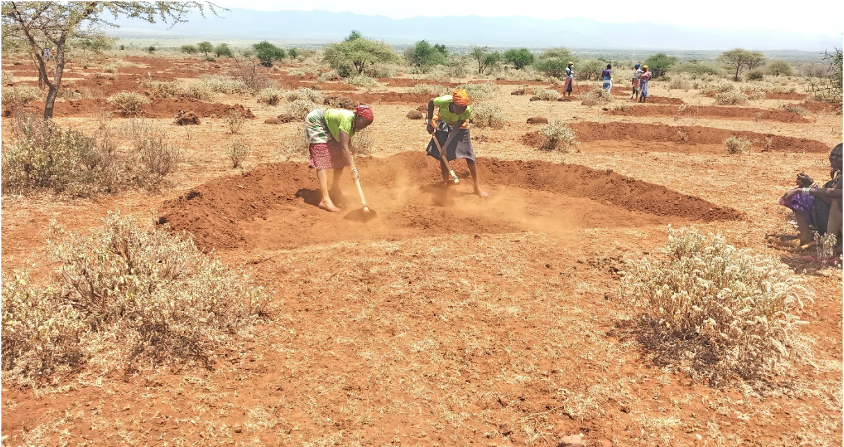
Figure 4: Bund digging in Ilchalai
